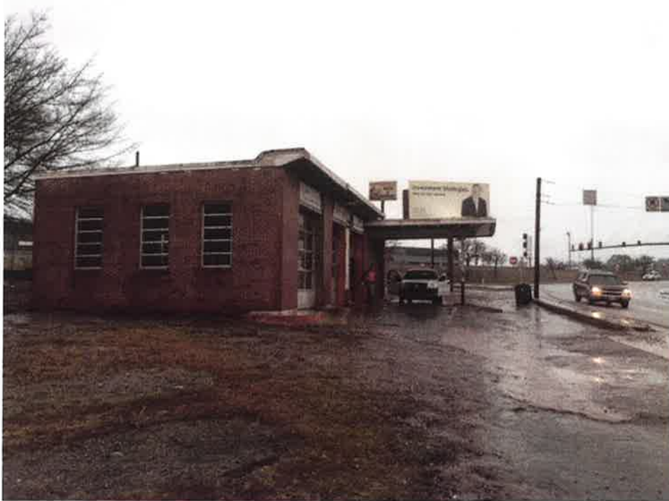
Photo No. 3 Description West side of building and parking lot Direction E Date December 23, 2015 Photographer S. Pfeifer
