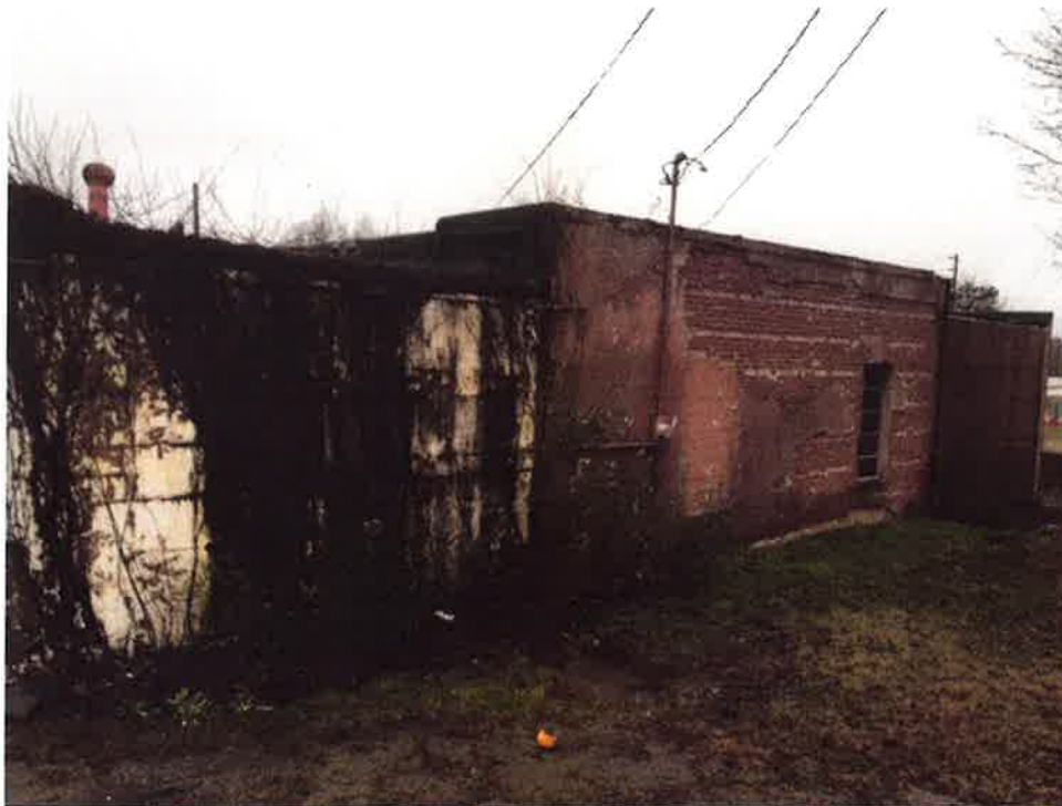
Photo No. 4 Description North side of building Direction SW Date December 23, 2015 Photographer S. Pfeifer
