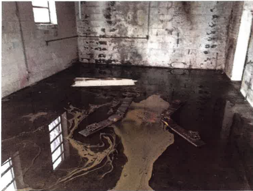
Photo No. 7 Description Garage bay #3 Date December 23, 2015 Photographer S. Pfeifer
