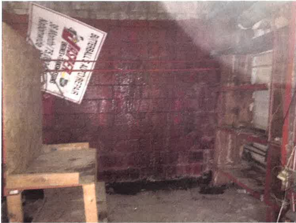
Photo No. 11 Description Office/storage room inside east side of building Date December 23, 2015 Photographer S. Pfeifer
