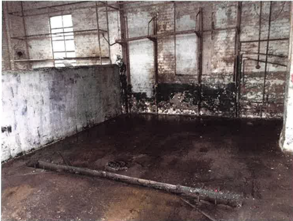
Photo No. 5 Description Garage bay #1 Date December 23, 2015 Photographer S. Pfeifer
