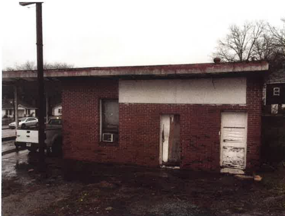
Photo No. 2 Description East side of building Direction W Date December 23, 2015 Photographer S. Pfeifer
