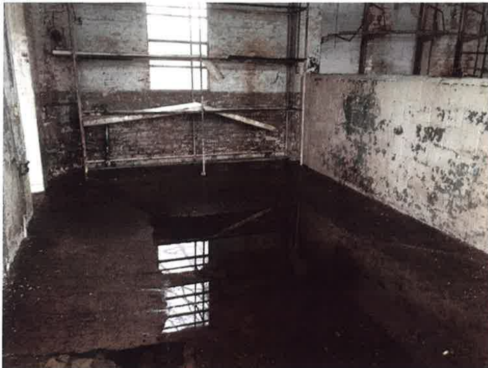
Photo No. 6 Description Garage bay #2 Date December 23, 2015 Photographer S. Pfeifer
