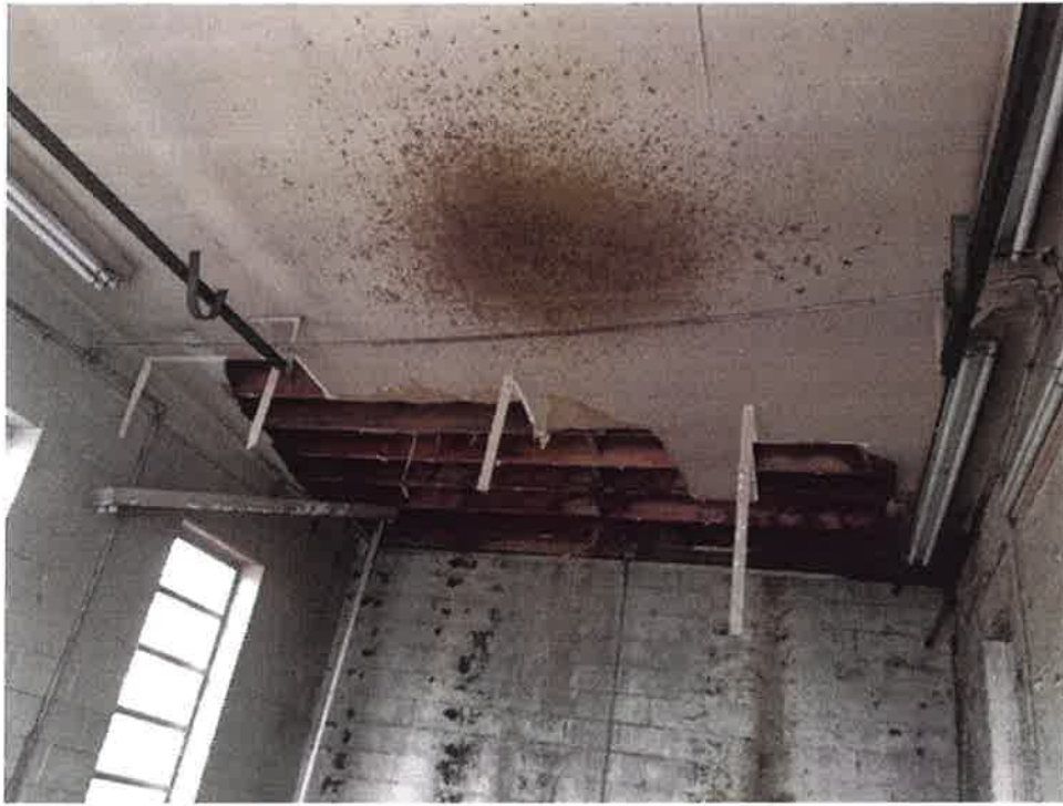
Photo No. 9 Description Ceiling above garage bay #3 Date December 23, 2015 Photographer S. Pfeifer
