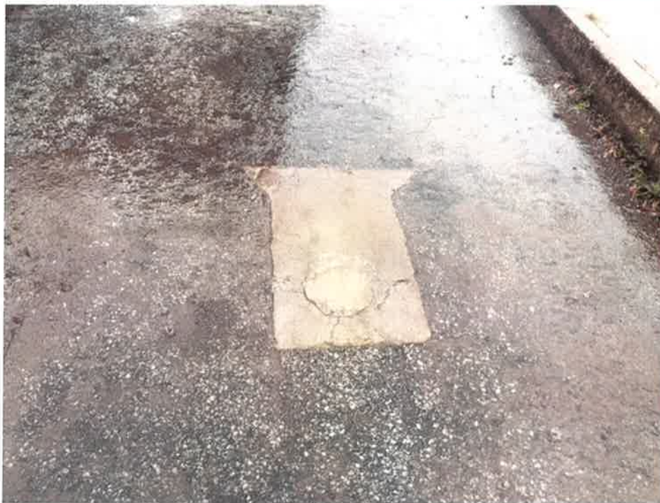
Photo No. 19 Description Possible former monitoring well in parking lot on south side of building Date December 23, 2015 Photographer S. Pfeifer
