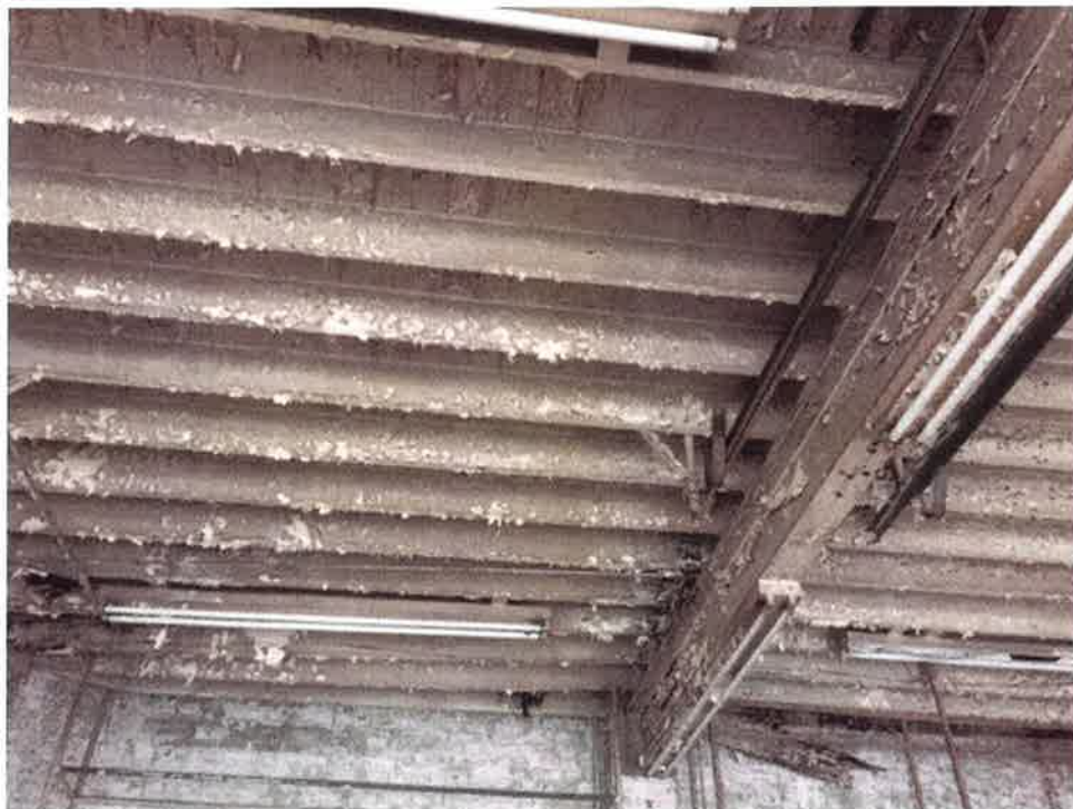
Photo No. 8 Description Ceiling above garage bay #2 Date December 23, 2015 Photographer S. Pfeifer
