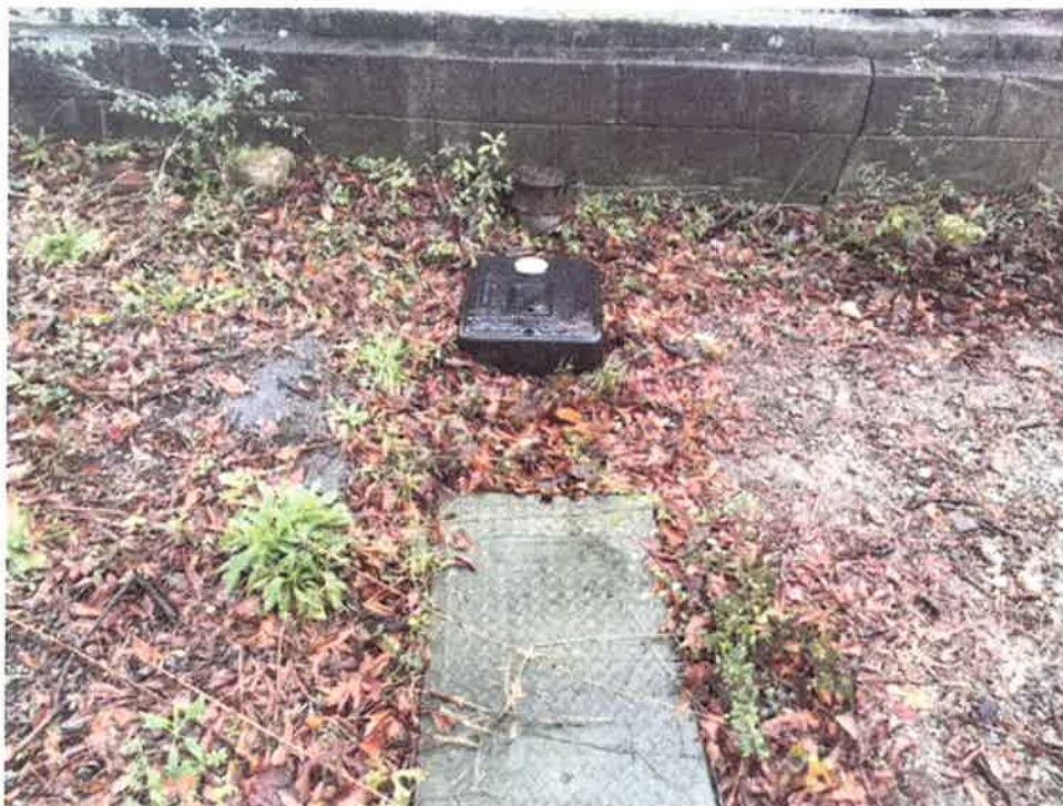
Photo No. 20 Description Water utilities in north corner of the property Date December 23, 2015 Photographer S. Pfeifer
