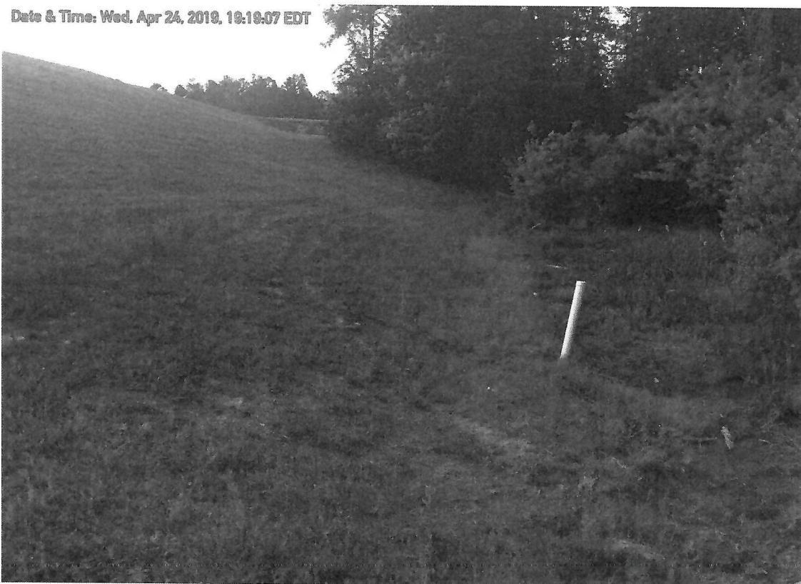
View facing northerly along downstream toe of Main Dam.
