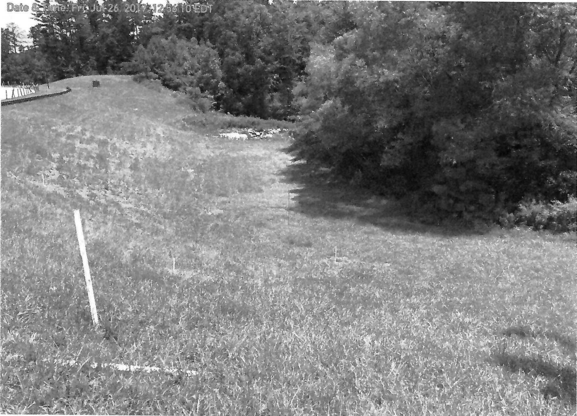
View facing northerly from right abutment of Saddle Dam. The embankment is dry. Six temporary observation wells were installed to determine the water level in the embankment/toe. (7/26/19)
