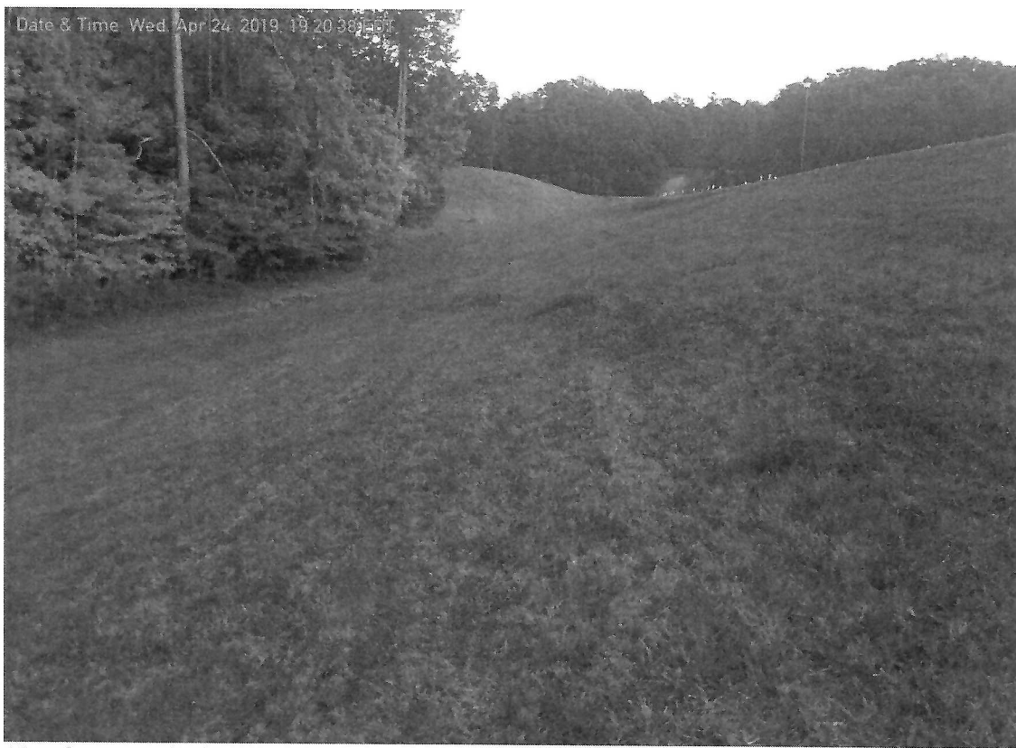
View facing southerly along mid-slope of Main Dam of irregular dam surface.
