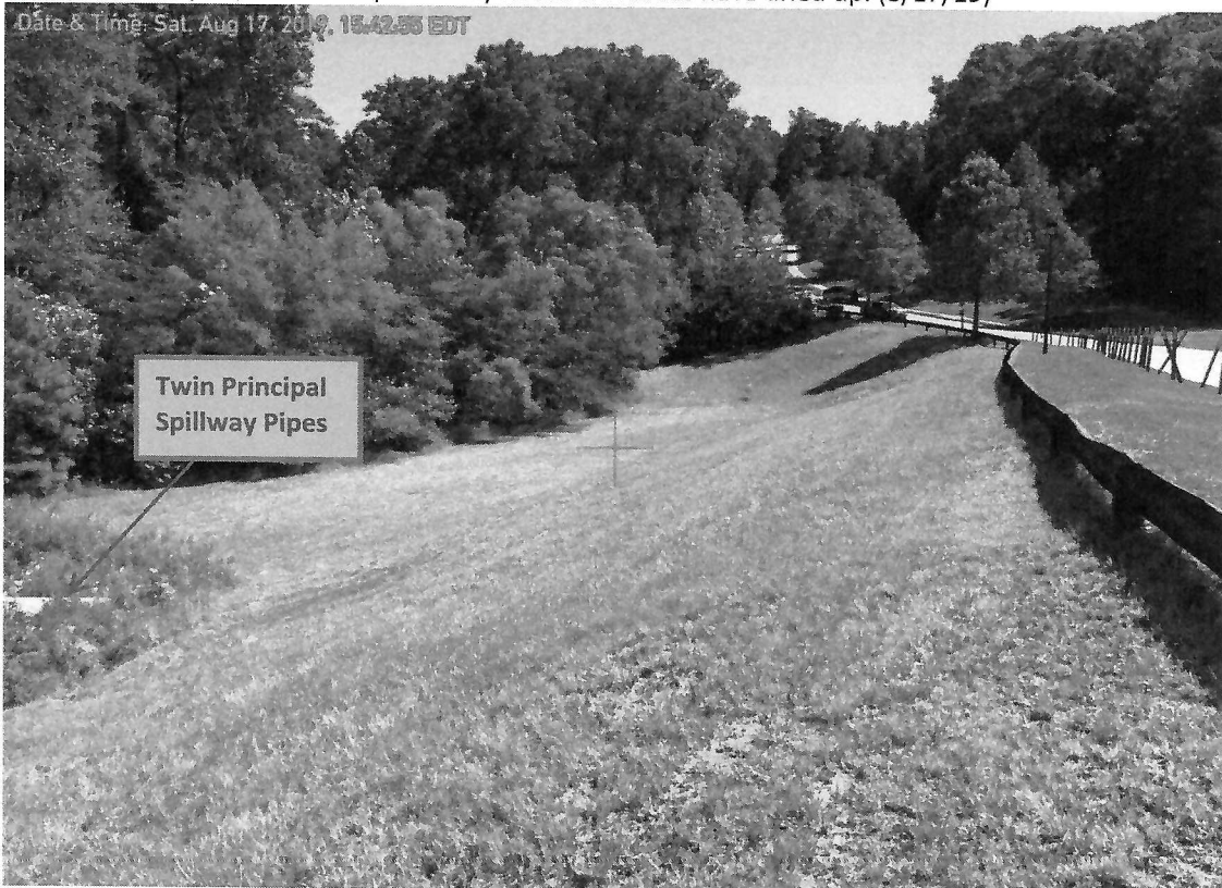
View facing southerly from left abutment of Saddle Dam. (8/17/19)
