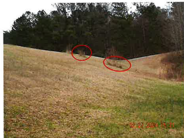
Looking left from right toe with small trees in line with principal spillway
