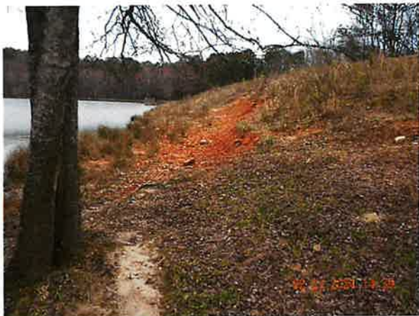
Looking left on right end of the dam at trees and eroded cow trails
