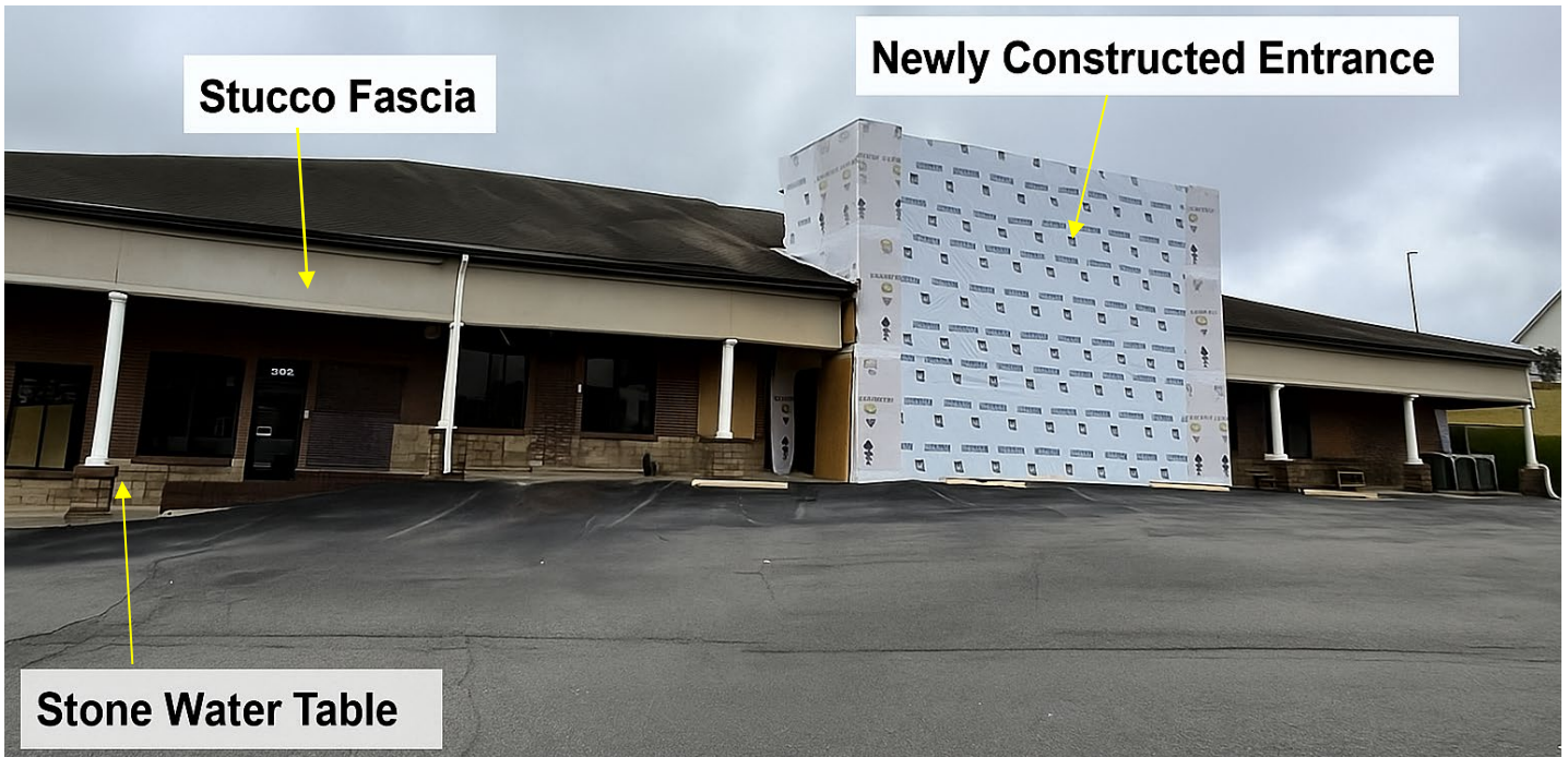
FIGURE 5. FRONT ELEVATION WITH FACADE ELEMENTS LABELED
