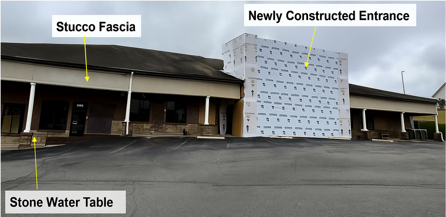
FIGURE 5. FRONT ELEVATION WITH FACADE ELEMENTS LABELED
