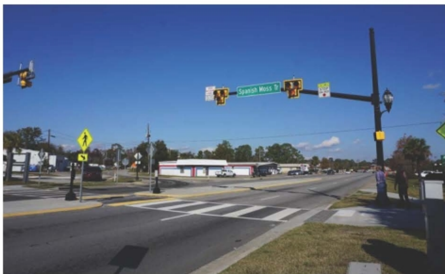
Typical trail at-grade crossing with a HAWK signal
