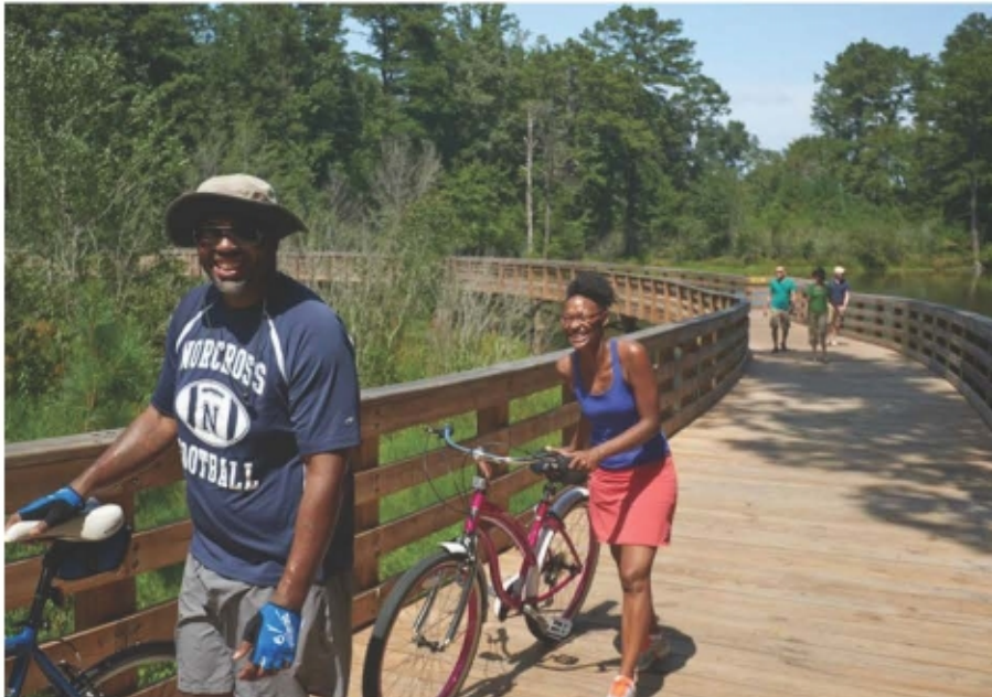
Boardwalk structure at Panola Mountain State Park
