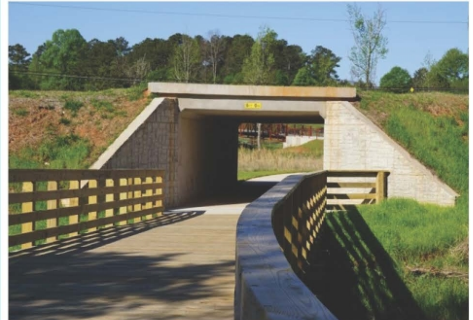
Box culvert structure allows trail underpassing under a roadway
