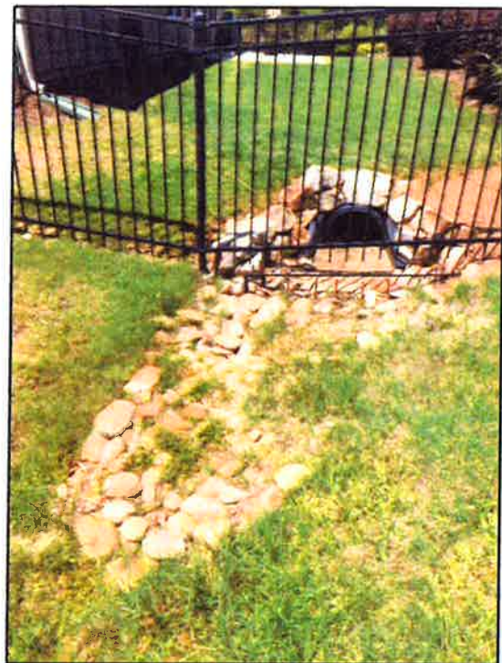
Photo 6: Northeast corner of lot 25, Culvert with riprap
