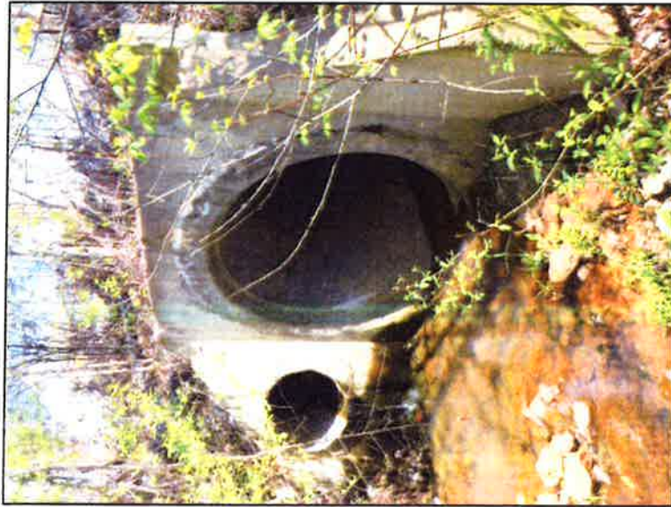
Photo 4: Perennial Stream 1 Culvert under Creekhead Road
