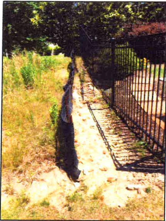
Photo 5: Southeastern corner of Lot 23. Riprap leading into a Culvert
