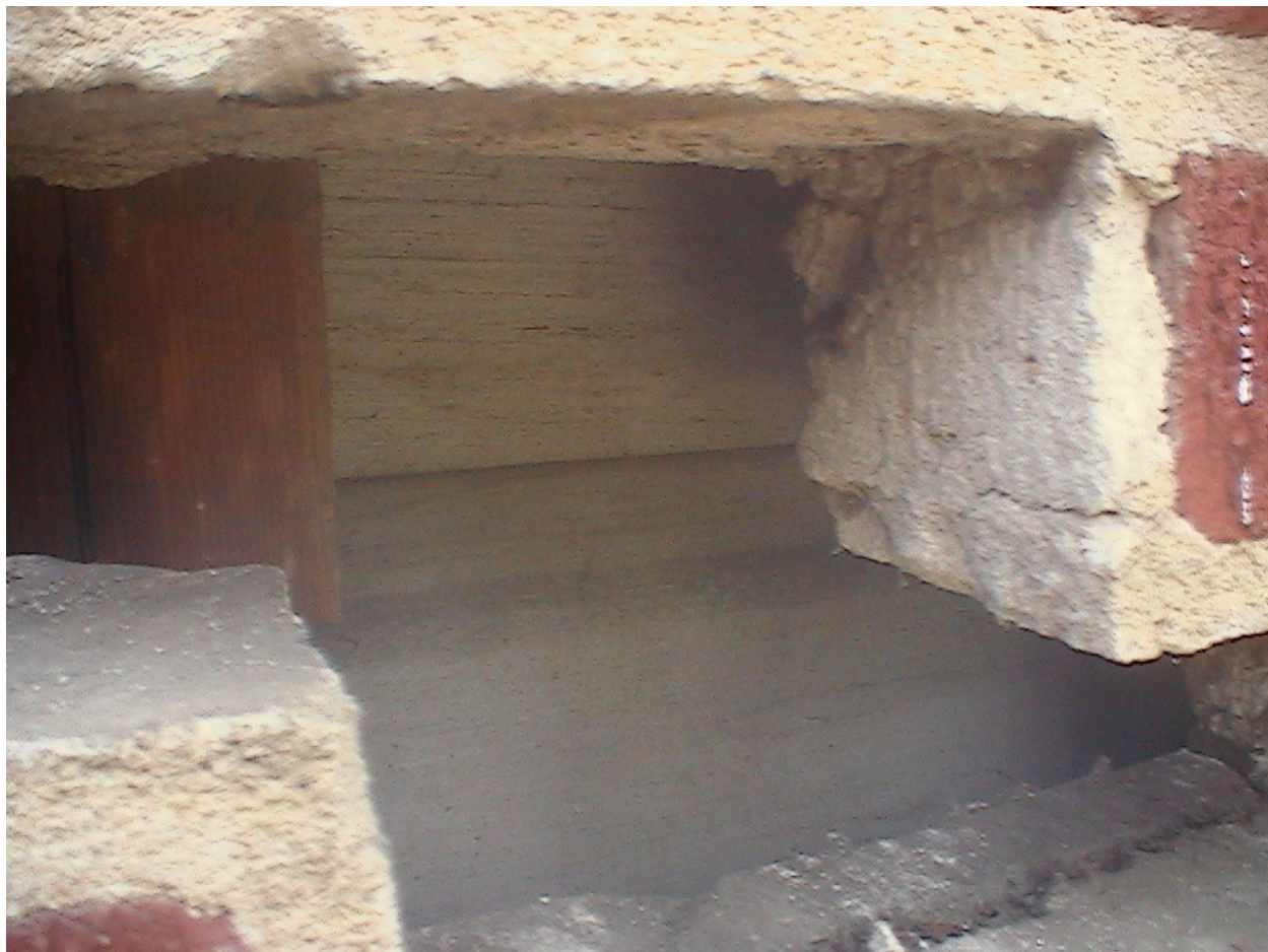
First Presbyterian Church Image 6 showing the 1885 wood sheathing under the 1930 brick sheathing (Photo by Ernest Everett Blevins; waymarking.com –retrieved 2-22-19)
