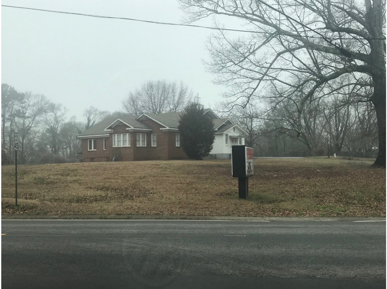
Villa Rica City Hospital 3 showing front/side (taken 2-22-2019)
