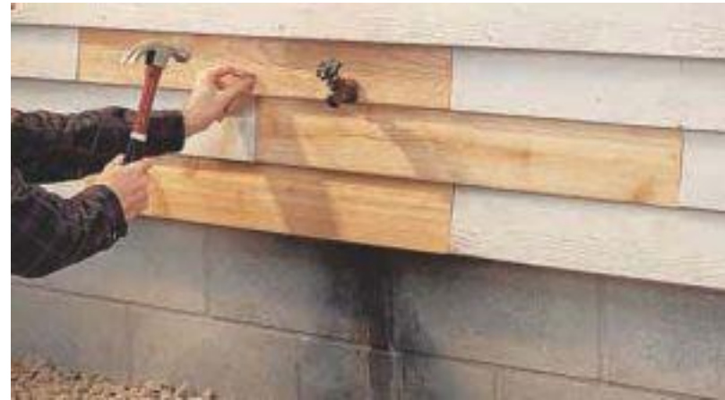
Siding should be repaired in-kind using the same materials and similar construction methods.
