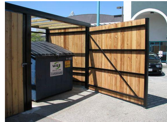
Dumpster facilities should be enclosed and out of view of the public.
