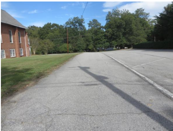
View along Dallas Road.
