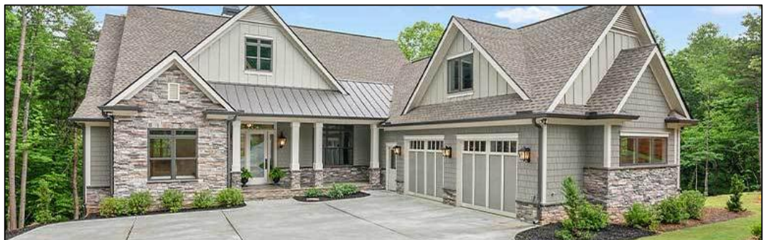
Above: Court- entry garage
