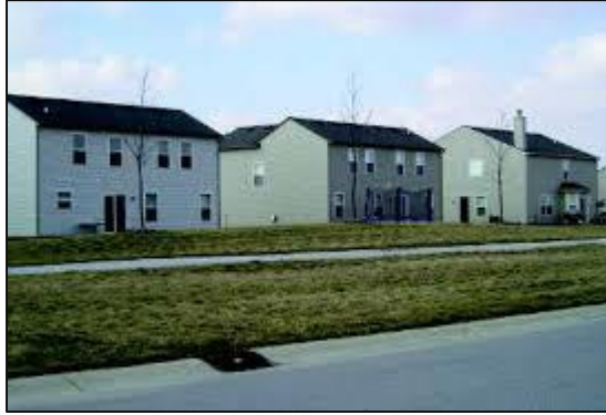
Above: The rear elevation of these residences lacks character as viewed from thoroughfares.
