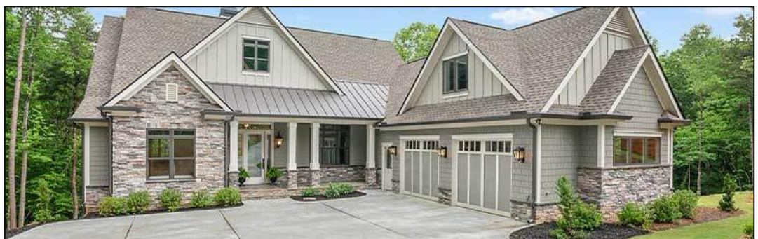
Above: Court- entry garage
