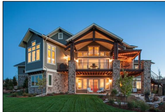
Above: Full first floor masonry wrap around exterior.
