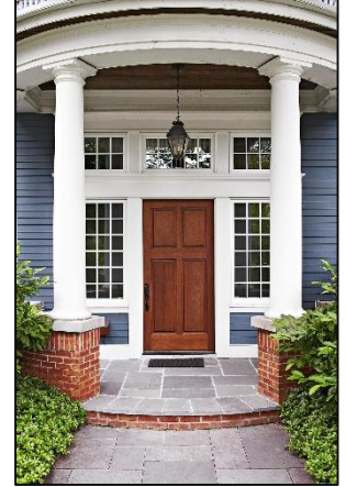
Above: Enhanced entry
